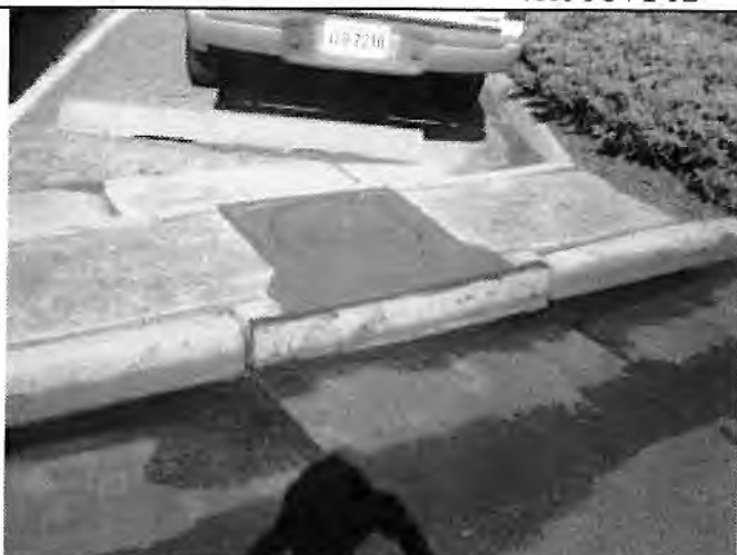
Photo 2. Curb inlet blocked off.
