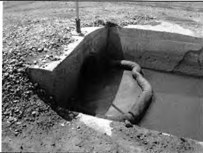
Photo 13. Oil boom in perimeter ditch.
