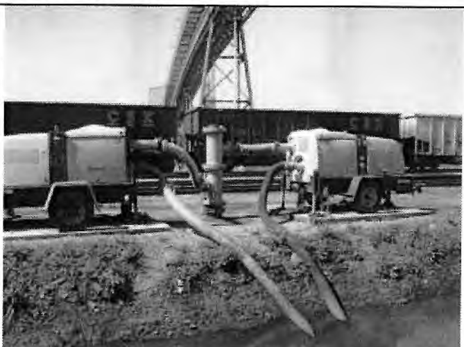
Photo 11. Pumps for transporting ditch water to the retention pond.
