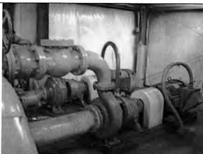
Photo 10. Discharge pump and rainbird pump.
