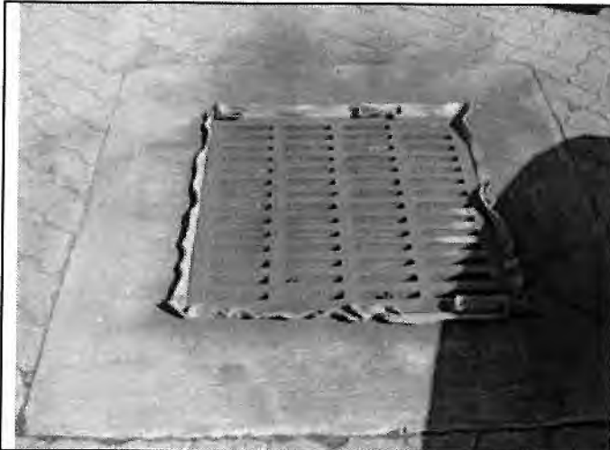
Photo 1. Drop inlet with filter cloth.
