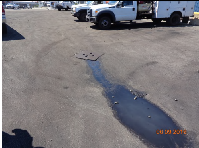
9) Water flowing to a drop inlet.
