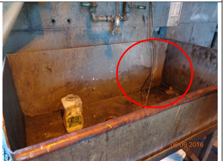
12) A small copper tube was discharging water to the sink with the sink connected to the pipe shown in #11. The source of the water was not determined at the time of the site visit.
