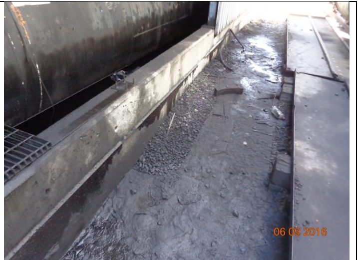
8) Tank labeled locomotive oil with the secondary containment structure almost filled. Oil was observed on the top and appears to be leaking out of the containment structure with a seam found between the two levels of the structure.
