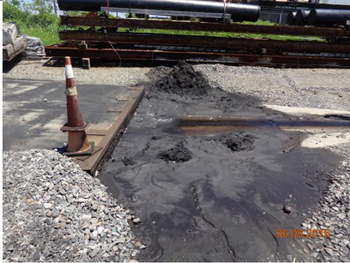
1) Pump station #4 with water running to the station. Coal fines are captured just prior to the pump station.
