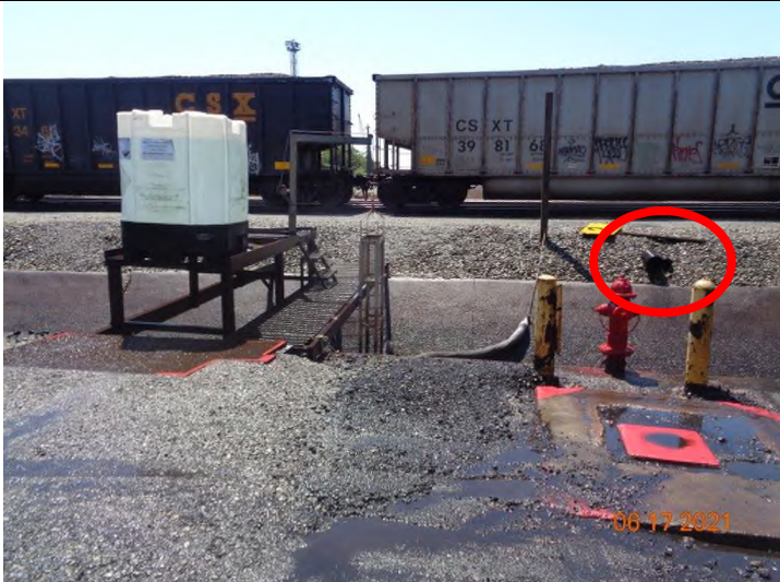
11) One of several NaOH containers placed in the facility for pH control. The circle shows two pipes that are not shown on the map. Multiple pipes are located in the ditch line that are not shown on the map.
