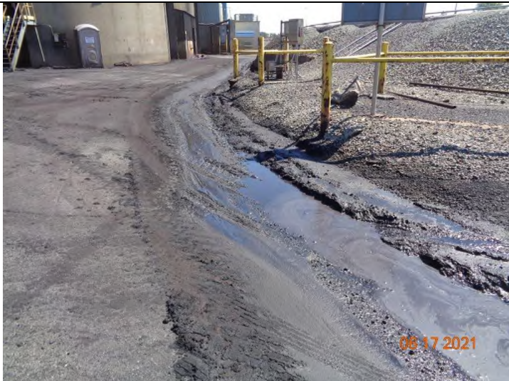
3) View to the north, southeast of the surge silos with coal fines collecting in the concrete swale with discharge to the catch basin shown in photo 4. Cleanup is needed in this area too.
