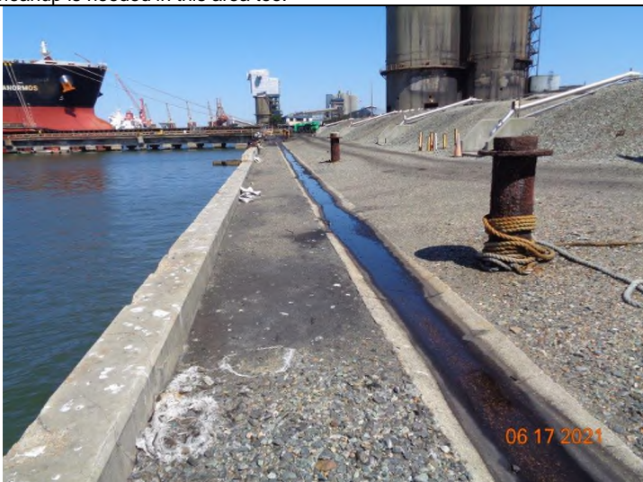
5) Swale along the bulkhead with pier 11 in the background. This drains to PS #3 that then pumps to PS #4 with discharge to Pond 1 or 3.
