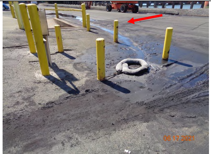
2) Drop inlet and (foreground) and trench drain (arrow) leading to PS #2. The inlet and the pump station is shown on the map, the trench drain is not shown on the map. Sweeping of the area is needed. Cleanup of solids was observed at another location.
