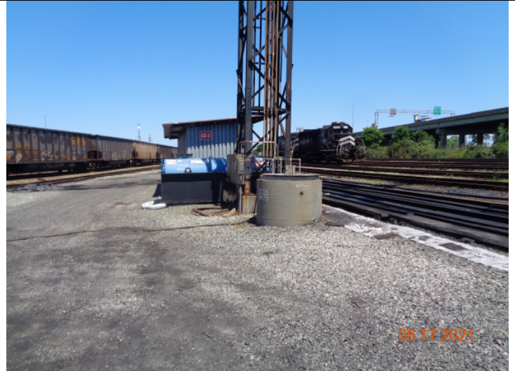
16) The building is CD 2 and the tank is ST 31. The spill pad shown in photo 14 is to the right. The iron support is the railcar dust suppression system that is not shown on the maps. The suppression system is shown in photo 18 too.
