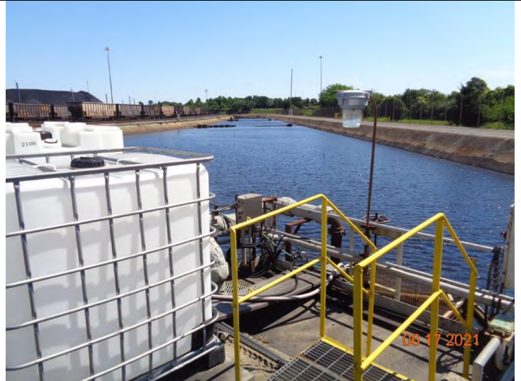
8) Pond 3, looking to the northeast. The containers have NaOH for neutralizing the pH.
