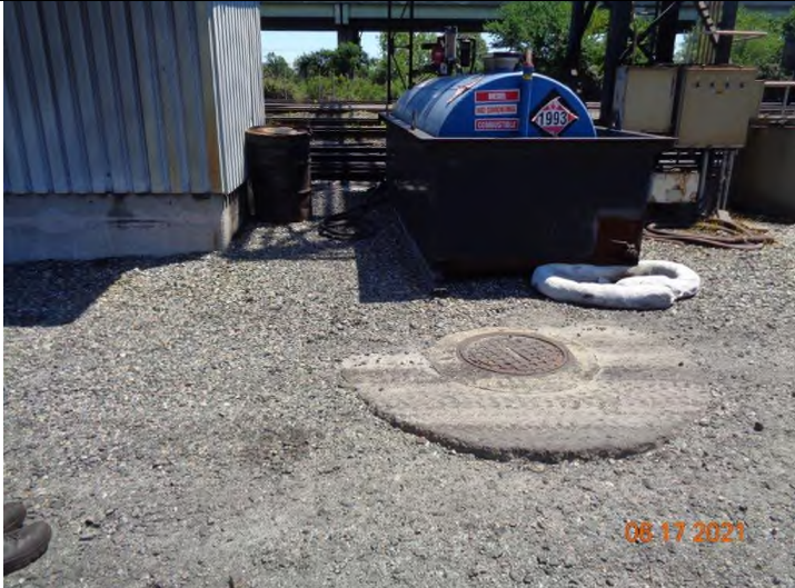
15) Oil water separator access. The blue building is CD-2 and contains ST (storage tank) -7. The storage tank shown above is ST-31. CD-2 is shown on the containment dikes map. ST-7 is not shown on either map.
