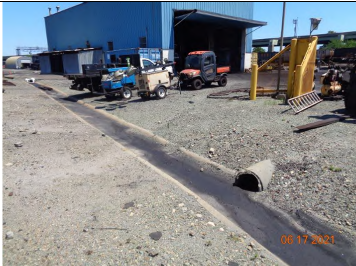
23) Maintenance building looking to the north. Concrete swale shown in 17-19 and 22 is in the foreground. An additional pipe from the northeast side of the building to the concrete swale is shown that is not included on the map.
