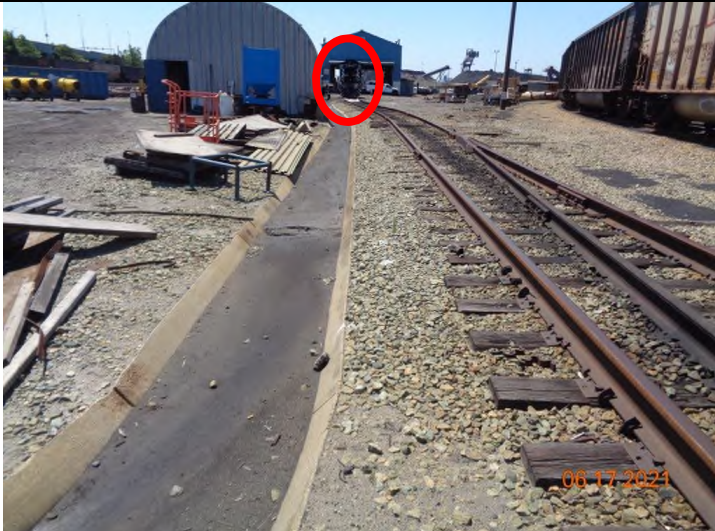
17) View to the south with the maintenance building in the background. The concrete swale and the Quonset style building are not shown on the map. This will connect to the main ditch system south of the maintenance building. The locomotive shown in 13 and 19-20 is circled.
