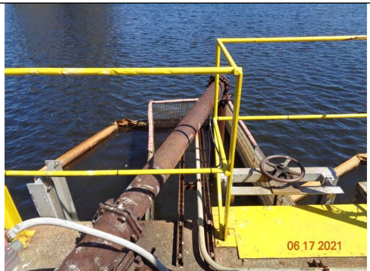
6) Pond 2 effluent piping with discharge to the outfall, shown in photo 7.
