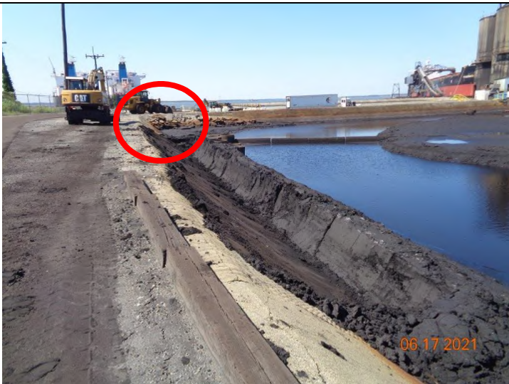
9) View to the southwest showing Pond 1. A pipe, circled, was observed near the southeast corner of the pond. This conveyance is not shown on the site map. Coal fines have been pushed together for eventual collection.
