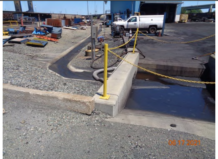
22) End of the concrete swale that started near CD-2 covered storage (See photos 17-19) The same truck circled in photo 21 is shown in this photos with that area a wash/rinse location.
