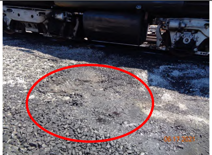
20) The circle shows areas where oil has either been spilled or seeped through the ballast.
