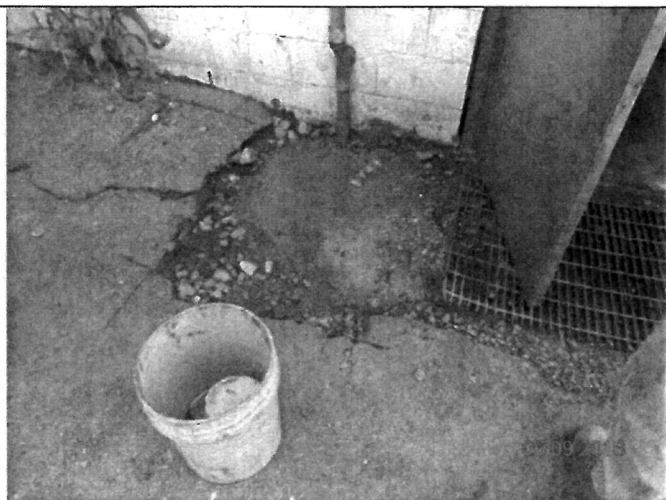
11) The pipe along the wall is broken open and leaking out on to the ground. This has since been fixed with the flow sent to the sanitary sewer.
