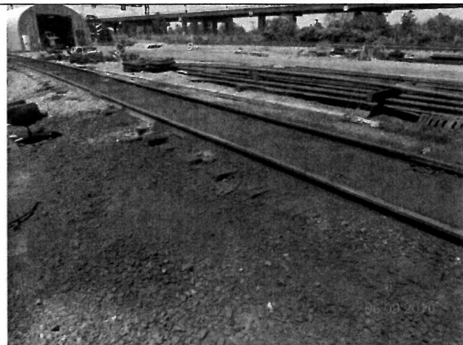
5) Railroad tracks with petroleum saturated area between the rails leaking to the ballast on each side of the track. This continues to the left and the building in the background.
