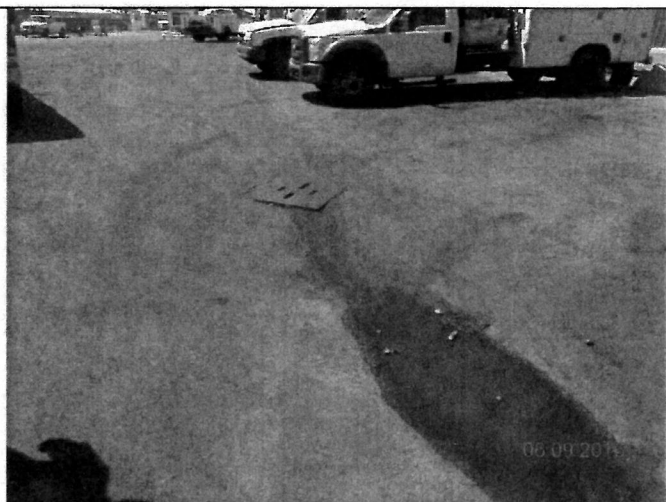
9) Water flowing to a drop inlet.
