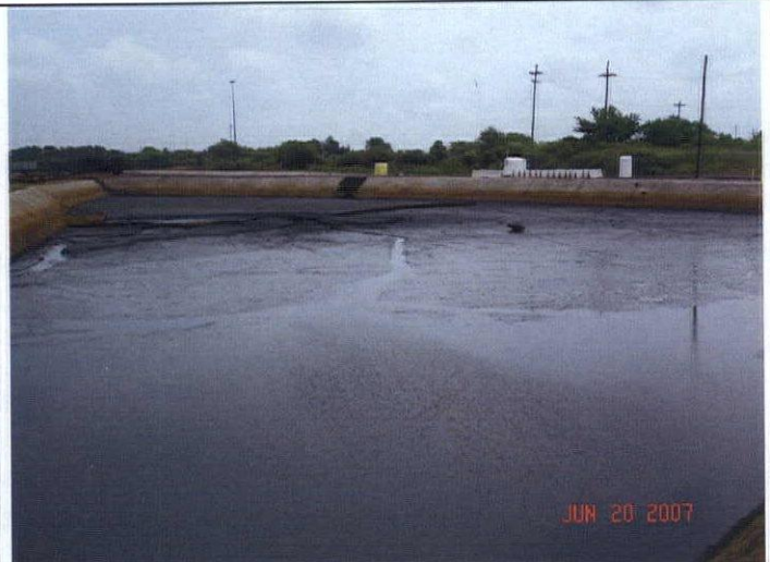
Pond #1 with coal fines that needs cleaning out. This pond and pond #3 are scheduled for cleaning.
