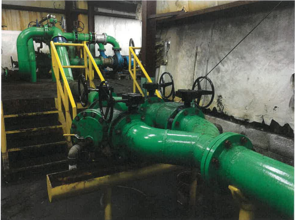
Pier IX utilizes parallel strainers so that system may be cleaned without taking the water supply out of service.
