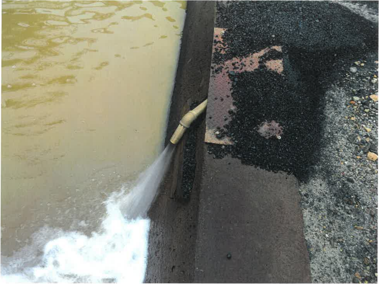
Pier IX continues to utilize a circulation line when pH corrections are needed to allow the circulation of pond water throughout the perimeter ditch-line.
