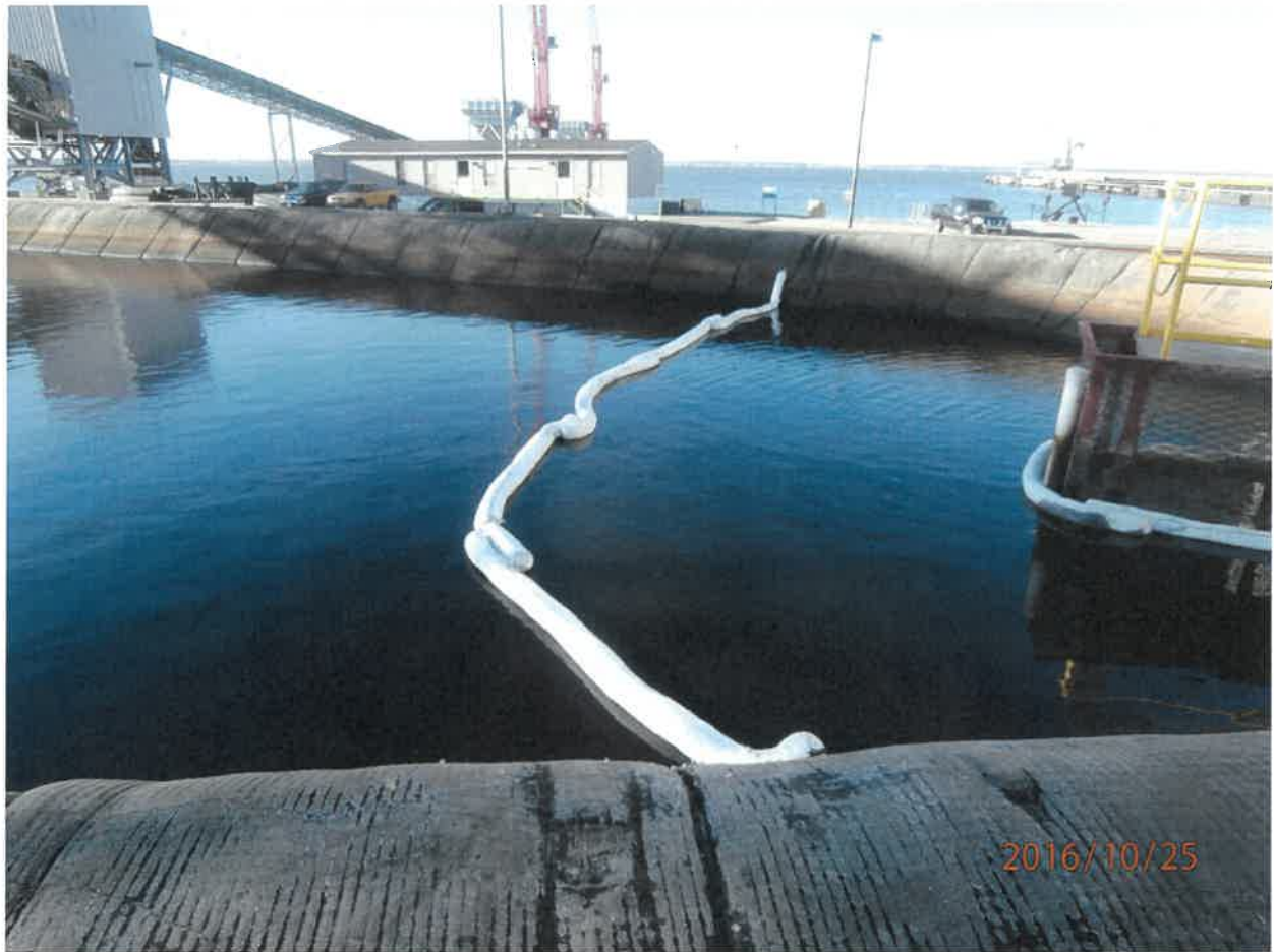
Oil booms in place at the retention pond stopping oil/debris from reaching outfall 001.
