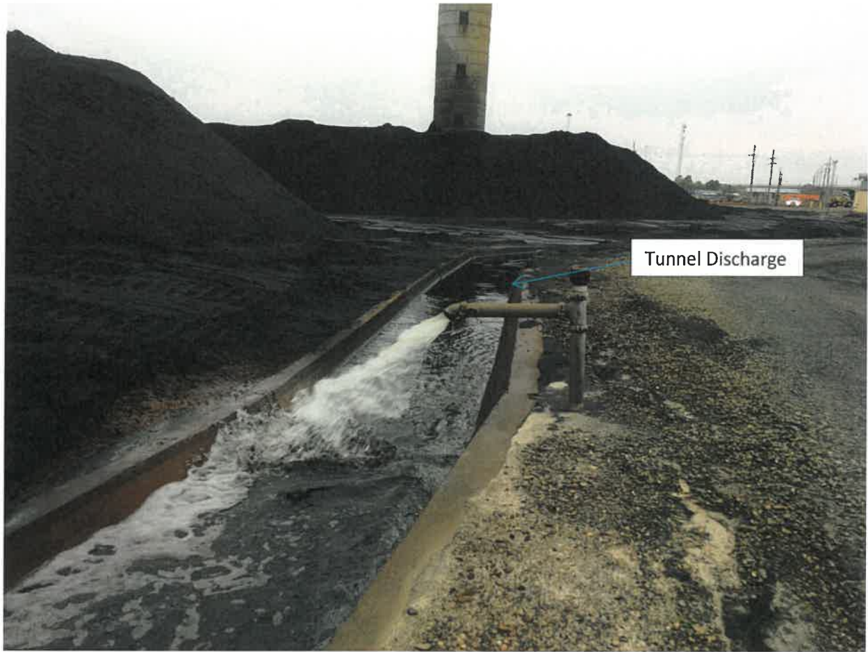
Pier IX pulls water from underground conveyor tunnels via submersible pumps and drains the water to the perimeter ditch-line.
