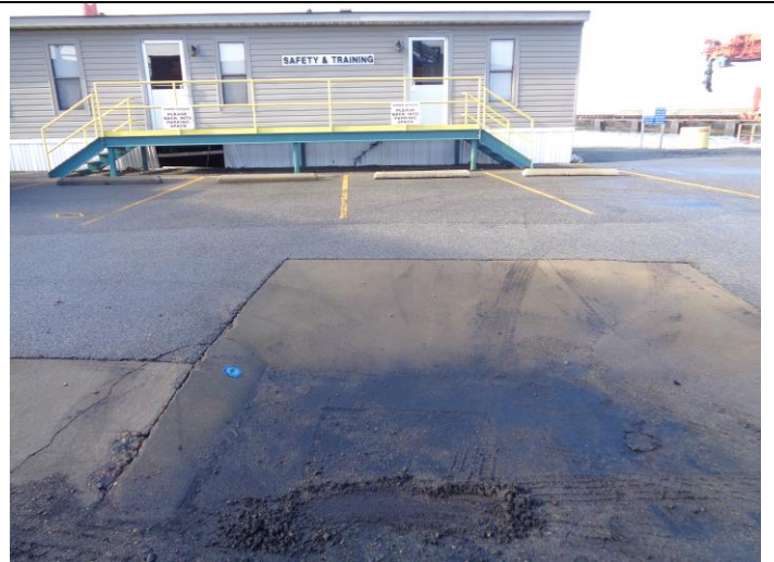
Photo 4. Another view of steel plate covering Outfall 003 drop inlet.
