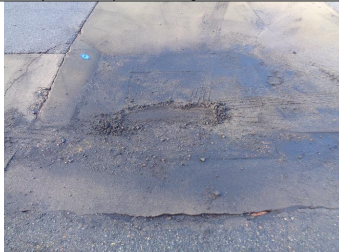
Photo 3. Buildup of solids overtop of covered Outfall 003 drop inlet.
