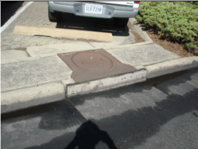
Photo 2. Curb inlet blocked off.
