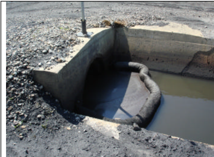
Photo 13. Oil boom in perimeter ditch.
