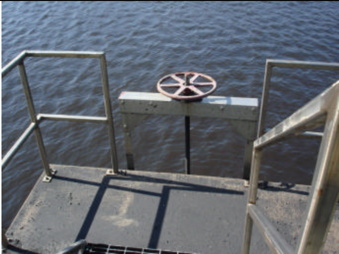
Photo 7. Gate for gravity flow from perimeter ditch to the retention pond.
