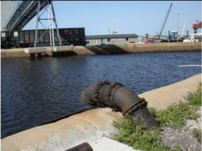
Photo 8. Discharge pipe for pumped discharges from perimeter ditch to the retention pond.
