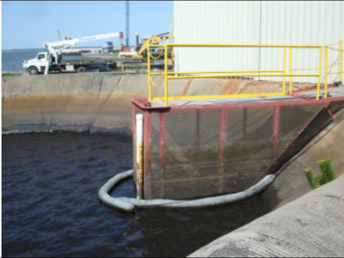
Photo 9. Pond outlet structure.
