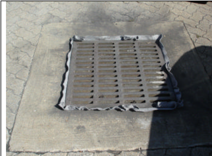
Photo 1. Drop inlet with filter cloth.
